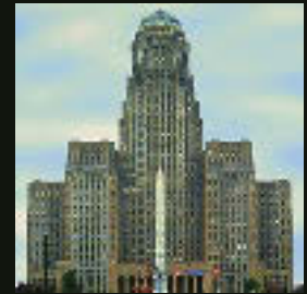
City Hall in Buffalo, New York, an Art Deco building.
