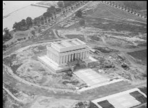
Lincoln Memorial under construction, 1919
