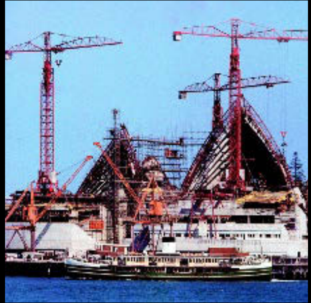
Sydney Opera House is a significant feat of engineering and technology involving ingenuity and creativity in many aspects of its design and construction. Photograph by Max Dupain and Associates
